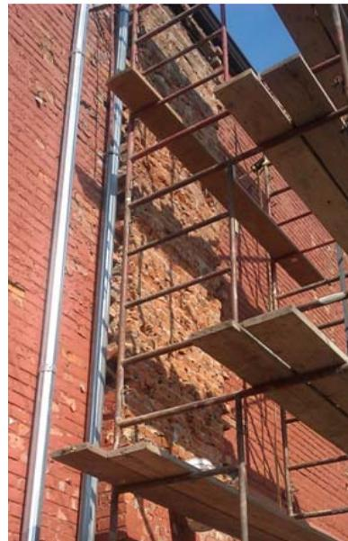
But after several days of tearing down the outside layer of brick and building it back up, it once again began to look like new. Followed by some stucco work and a new paint job, no one would have ever suspected it was in such bad disrepair. To the left is the pilaster with outer layer being removed.
